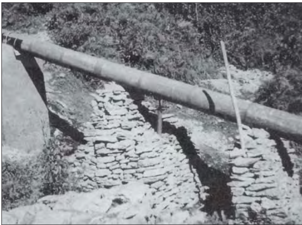
Photo 6.15 Temporary support for site welding work, jhankre mini-hydro, Nepal
