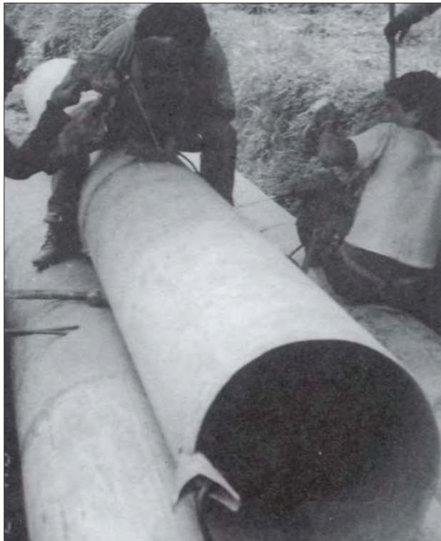
Photo 6.10 Site welding of penstock pipes, Jhankre mini-hydro
