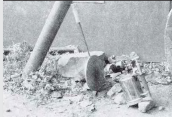
Photo 4.20 Heating the welding plate
