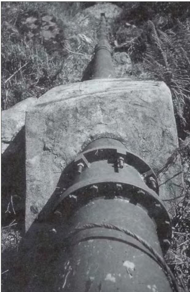
Photo 6.12 An expansion joint should be located just below an anchor block to protect the block from forces which it may not be designed to resist (Siklis)
