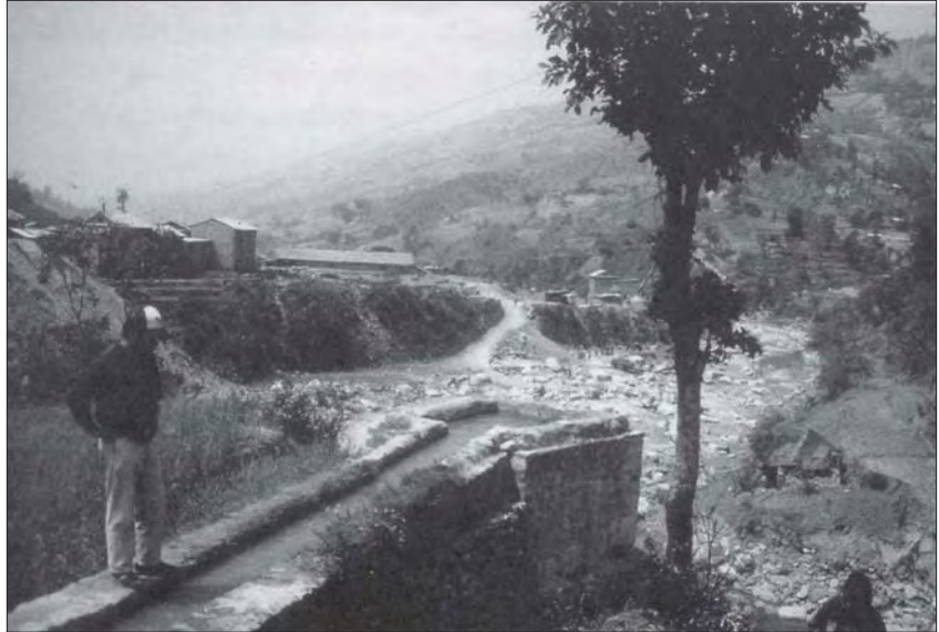
Photo 5.10 A cement masonry channel and forebay at the top of a steep slope (Dhading)
