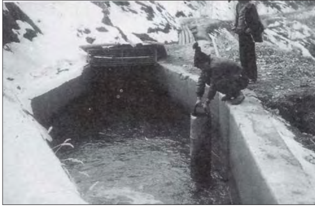
Photo 5.5 Settling basin at Jharkot
