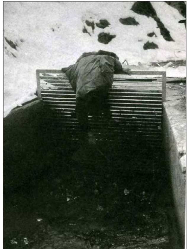
Photo 5.11 Cleaning can be difficult with horizontal bars
