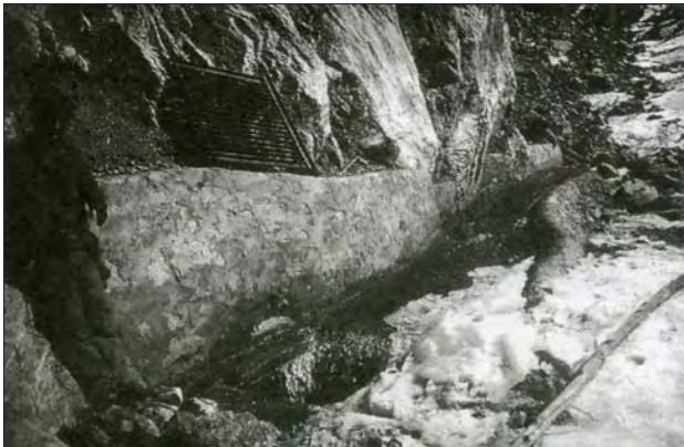
Photo 3.10 Bottom intake with the grill removed (Jhong)
