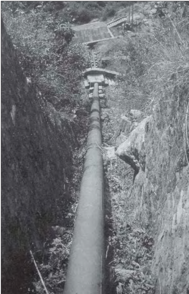
Photo 6.3 Excavation to reduce the cost of the penstock and reduce the need for anchors (Siklis)
