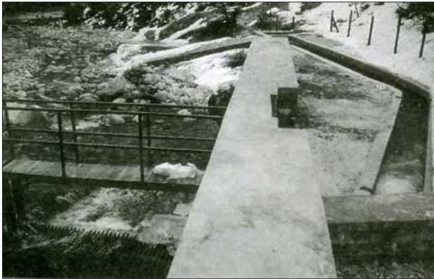
Photo 3.9 Bottom intake of Theme micro-hydro scheme, Nepal .
