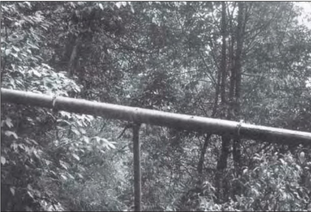
Photo 4.15 Jhankre mini-hydro headrace crossing Ghandruk, Nepal.
