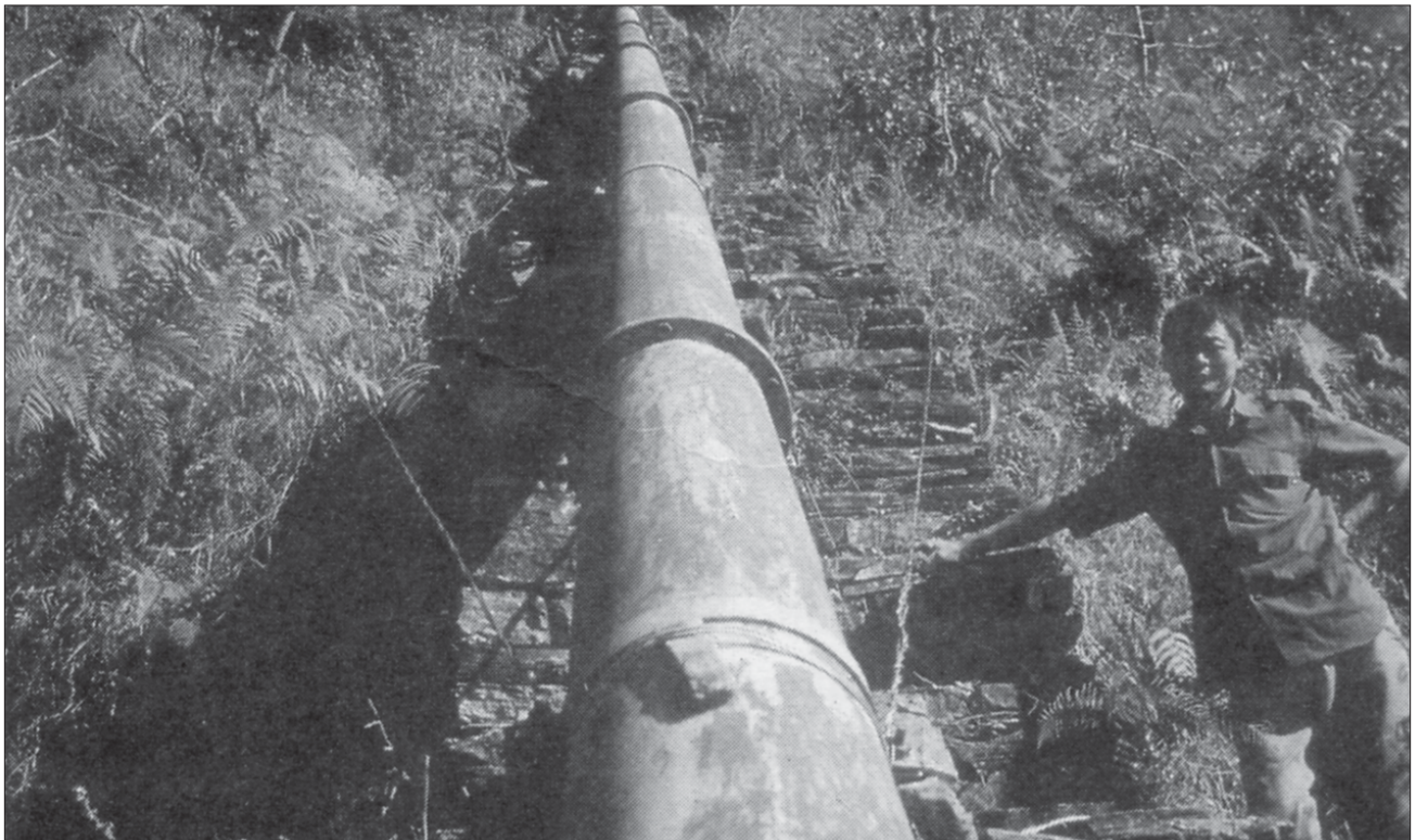
Photo 9.4 Stone masonry can provide slope stabilisation along the route of the penstock (Barpak)
