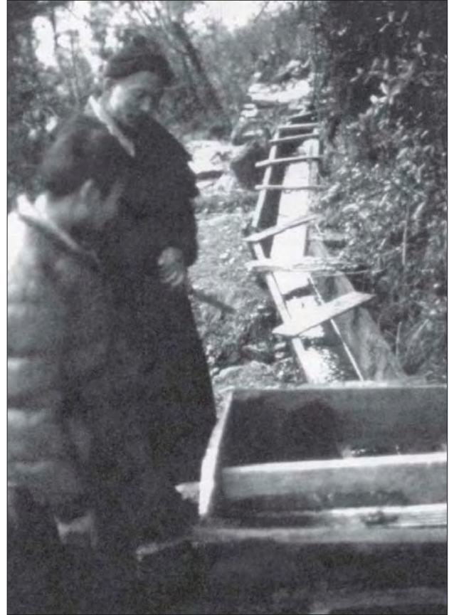
Photo 4.6 Timber canal with bracing supporting the sides, Thuptenchuling.
