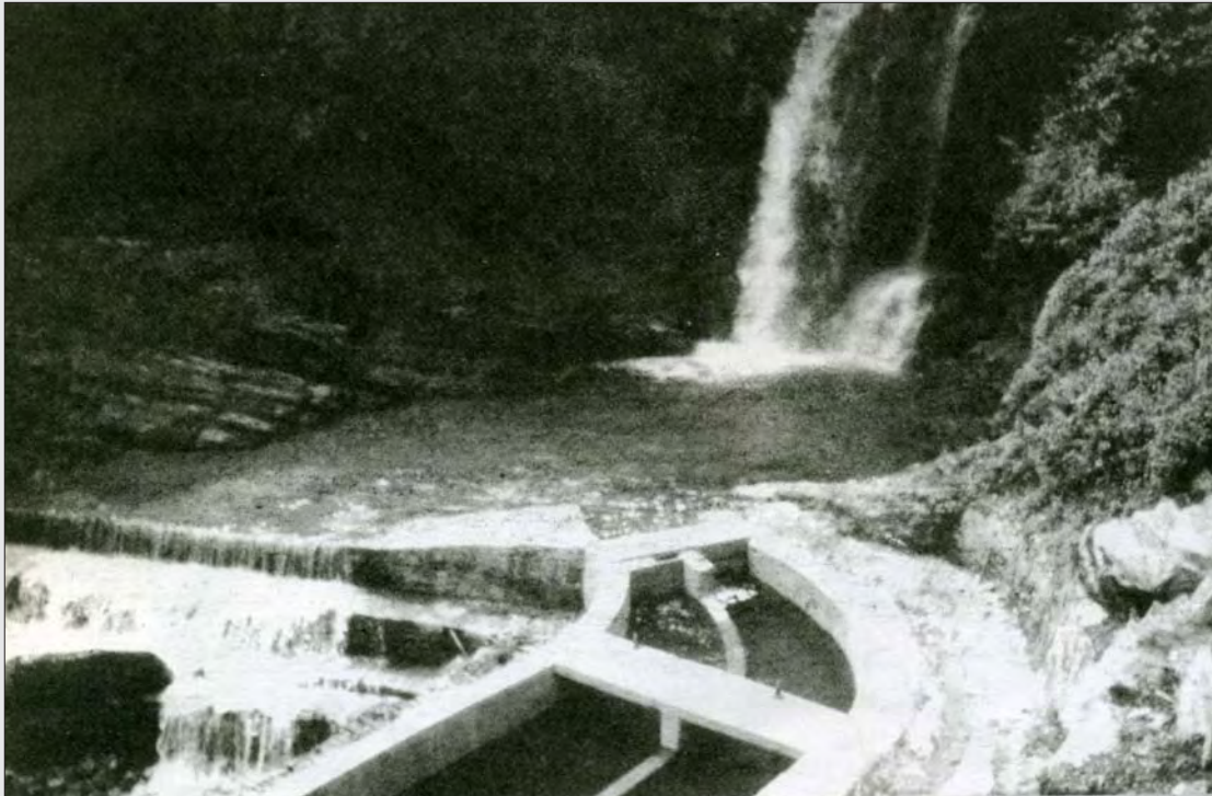
Photo 3.7 Diversion weir of the Jhankre Mini-Hydro Scheme
