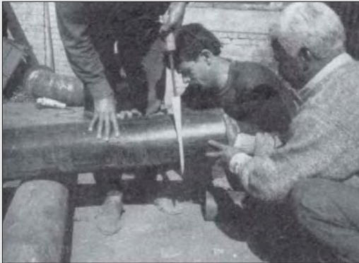
Photo 4.21 Joining HDPE pipes by pushing them while hot. Notice the Teflon bag.
