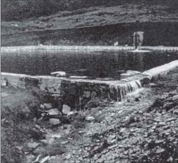
Photo 5.15 Ghandruk peaking reservoir after construction
