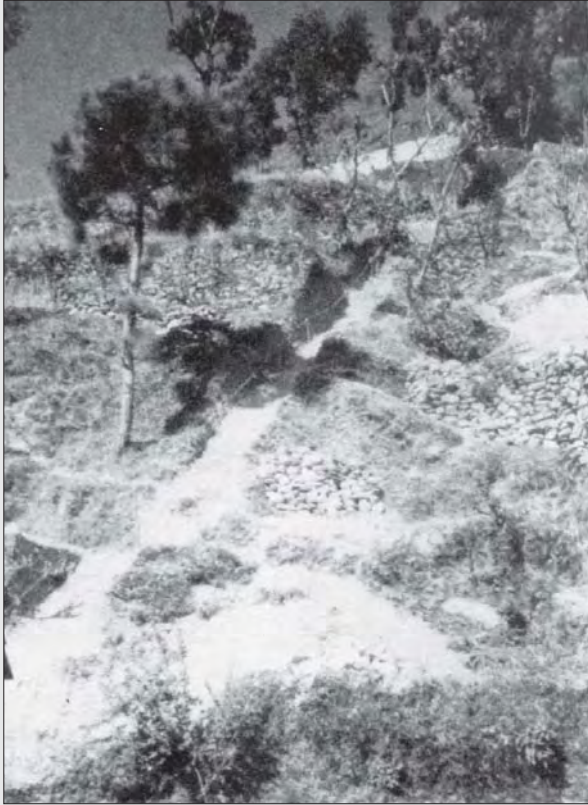
Photo 6.7 Excavation for penstock alignment, Galkot
