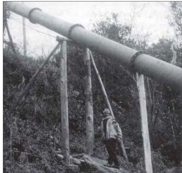
Photo 7.7 Wooden support piers at Kamche micro-hydro, Nepal
