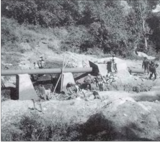
Photo 7.5 Stone masonry support piers, Jhankre mini-hydro scheme
