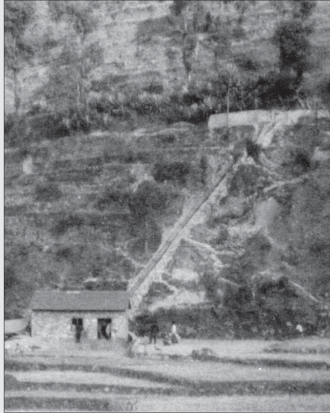
Photo 6.8 Penstock alignment, Galkot
