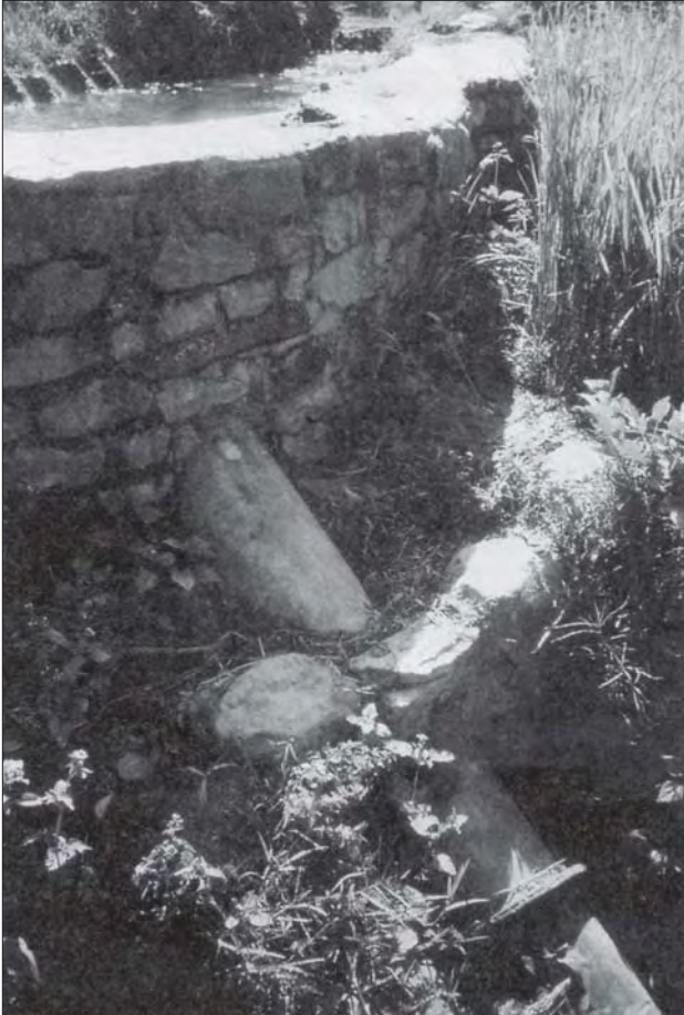
Photo 5.9 A dry stone masonry forebay showing the connection with the penstock
