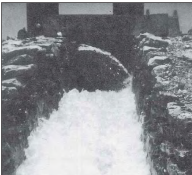
Photo 8.5 Tailrace channel of the Salleri Chialsa mini-hydro scheme
