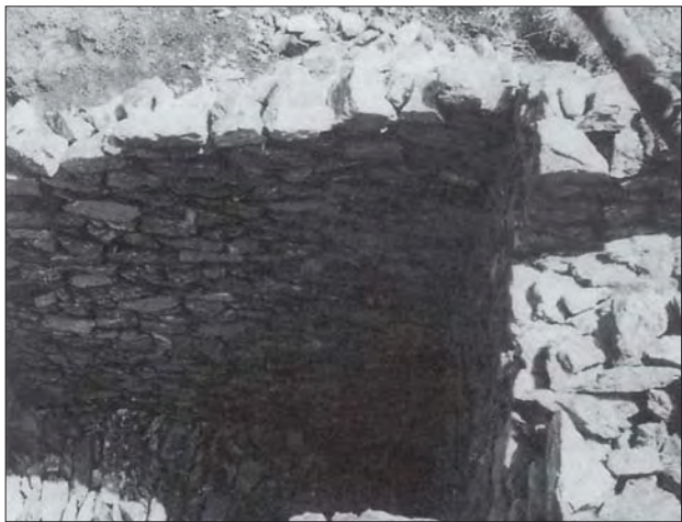
Photo 7.4 Use of dry stone wall for forework, Jhankre mini-hydro
