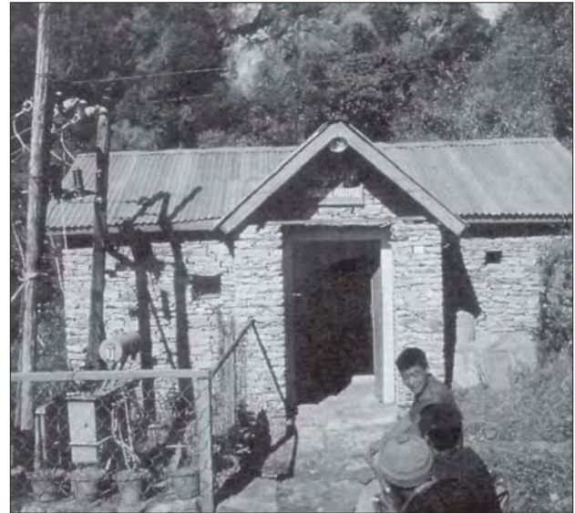
Photo 8.1 Powerhouse of the Barpak mini- hydro scheme
