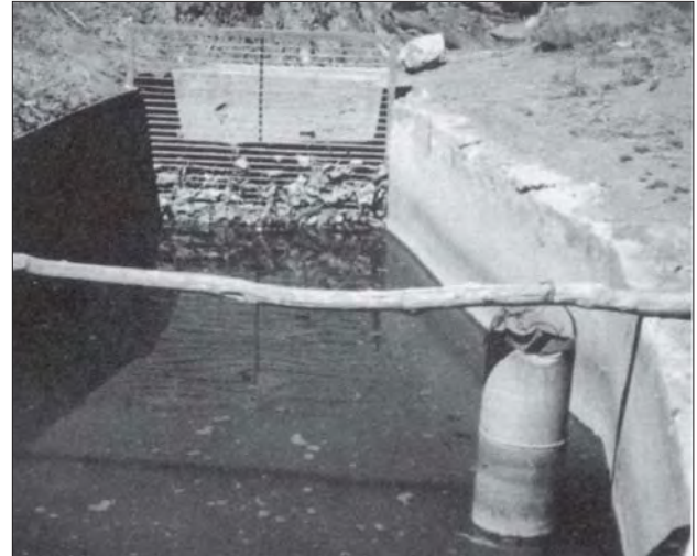
Photo 5.4 Jharkot settling basin
