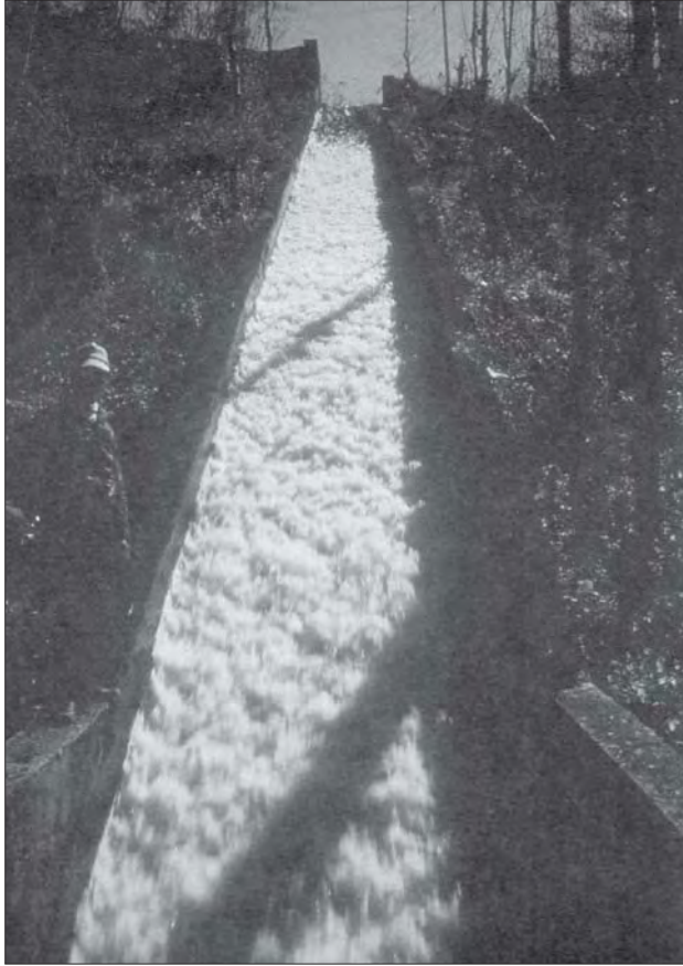
Photo 8.6 Tailrace channel of the Jhankre mini-hydro scheme
