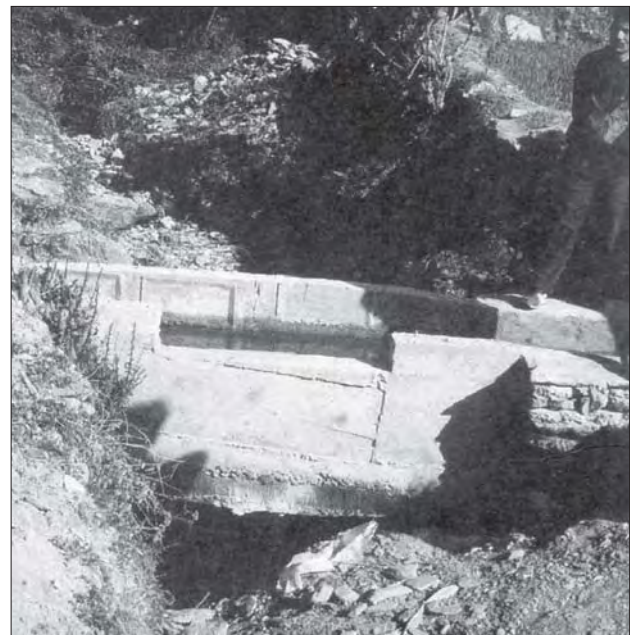
Photo 4.12 Spillway on a crossing where the excess flow is discharged into a gully, Galkot micro-hydro scheme, Baglung, Nepal.
