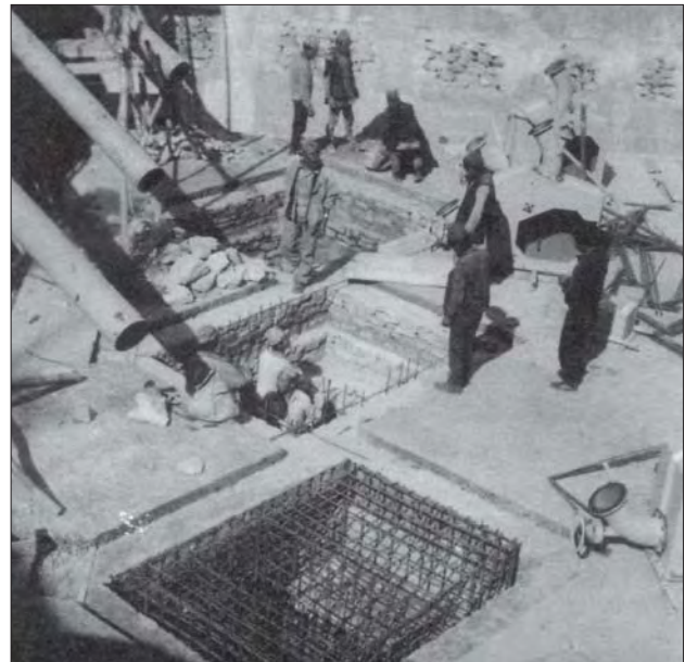
Photo 8.4 Construction of Jhankre mini-hydro machine foundation.
