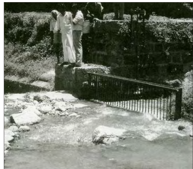
Photo 3.3 Where an intake is liable to attract floating debris a trashrack may be necessary ( Sri Lanka )
