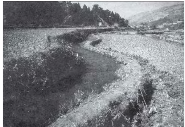
Photo 4.1 Earth Channel (Dhading)
