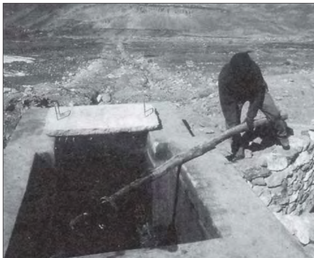
Photo 5.3 Lifting the flushing mechanism (Jhong)
