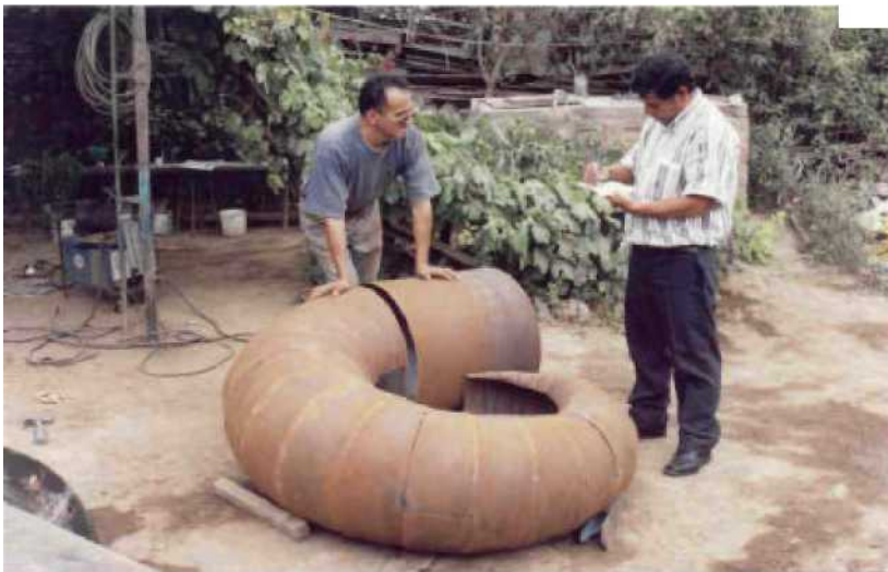
Figure 12: Welding of the spiral segments
