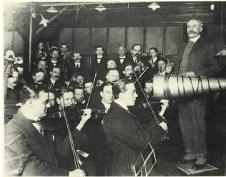
Fig 9.2 The composer Edward Elgar making a mechanical recording with an orchestra. The horn from the cutter can be seen on the right.
