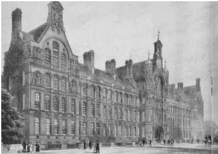
Fig 5.3 City and Guilds College Waterhouse building
