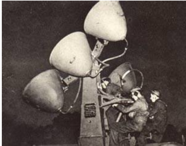
Fig 17.1 A team operating a sound locator
