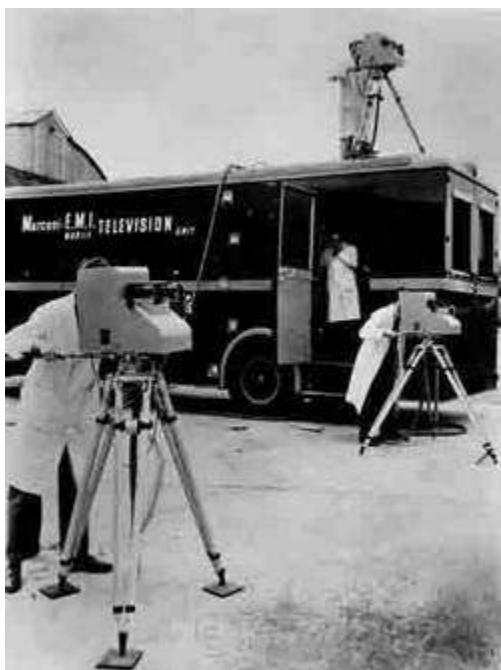
Fig 16.2 The outside broadcast unit with its three cameras that could operate up to 1000 ft from the truck
