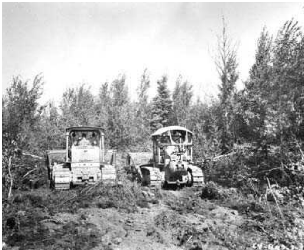
Construction on Hanson Lake Road, circa 1958.
