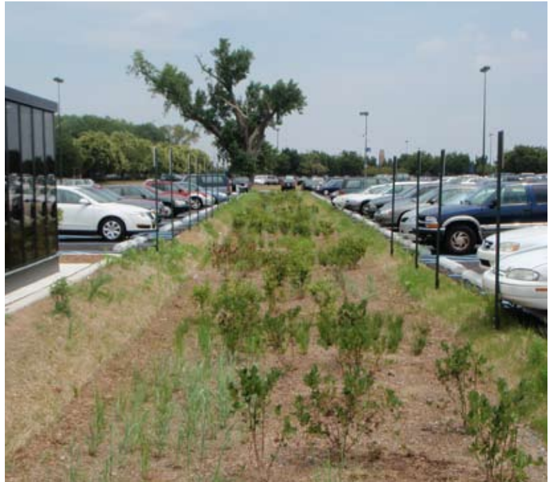
Above: A vegetated swale collects and infiltrates stormwater from an employee parking lot at the Philadelphia International Airport in the Schuylkill Watershed.
