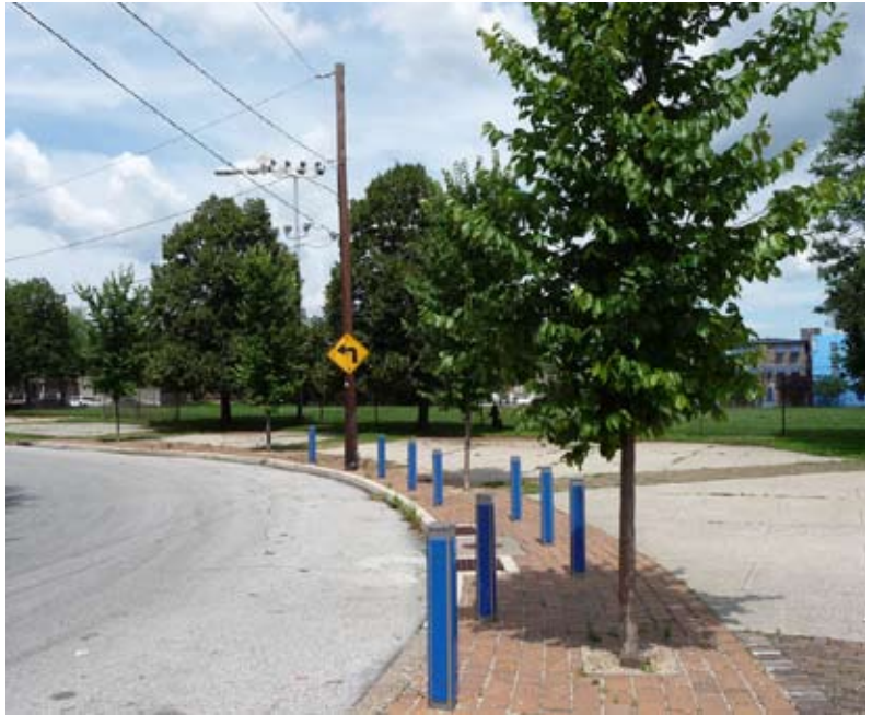
Above: The West Mill Creek Green Streets demonstration project in the Schuylkill Watershed includes a tree trench, permeable pavers and modified street inlets to divert stormwater into a subsurface infiltration bed.
