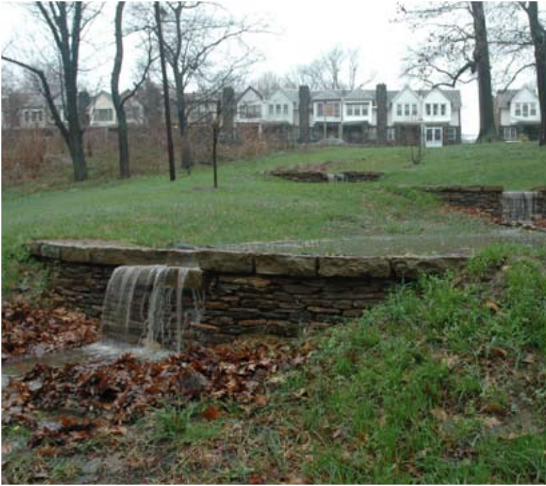
Above: The stormwater demonstration project at Cliveden Park captures runoff from adjacent streets and uses the park’s natural topography to detain and infiltrate stormwater in the Tookany/Tacony Frankford Watershed.
