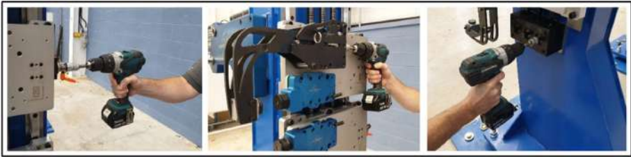
Fig. 11. Manual adjustment of the VADIS fixture with use of common power tools
