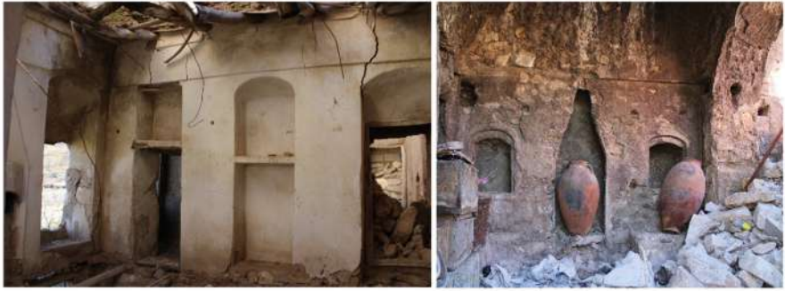
Fig. 4. Doors and windows transformed to wall niches used as shelves, cupboards or fire places.
