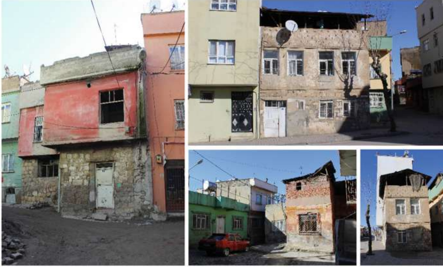
Fig. 9. Some examples of the cas houses in Siirt city center which are lost their original and authentic form and properties.
