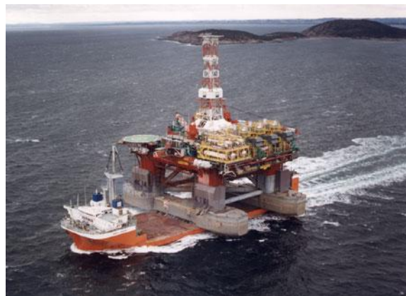
Figure 5.4.: The Petrobras P-36 oil platform.
