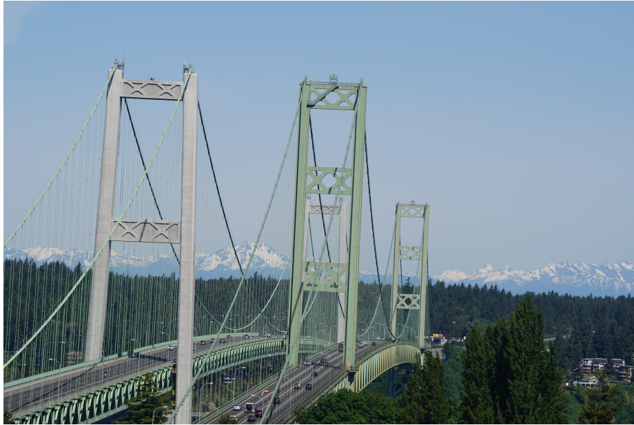
Figure 4.4.11: The Tacoma Narrows Bridge (2017)
