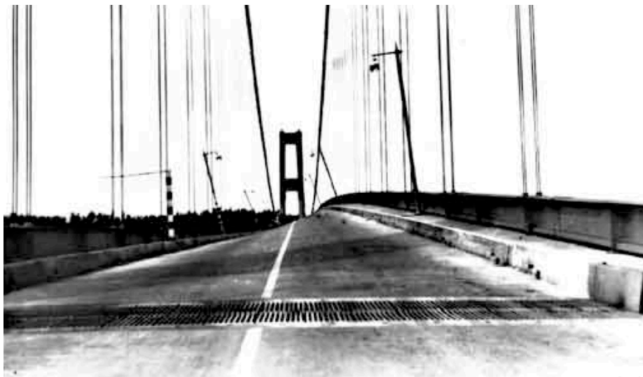
Figure 4.4.10: The Tacoma Narrows Bridge
