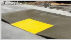
A sidewalk ramp
