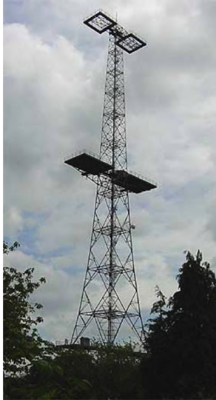
Figure 14-12 Chain Home Radar Station
